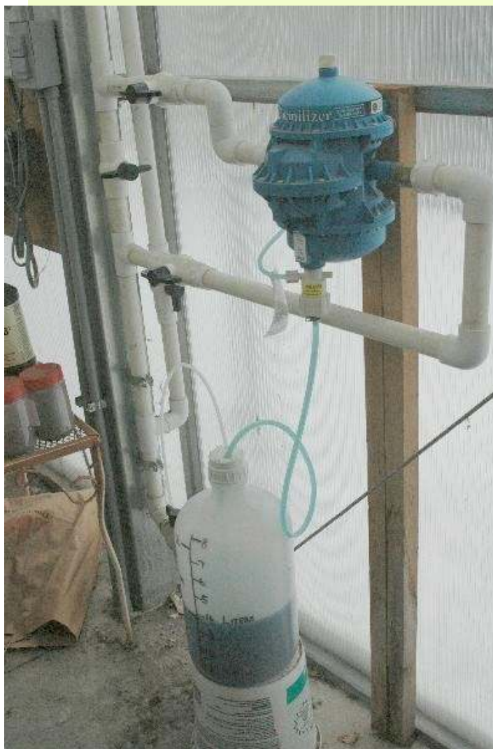
Jim's automated, drip-irrigation fertilization system at work in his large Clivia House. Photo by Jim Shields.
